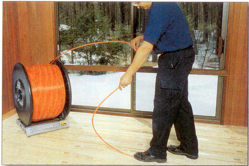
Installation of a hardwood floor over the radiant subfloor panels.
